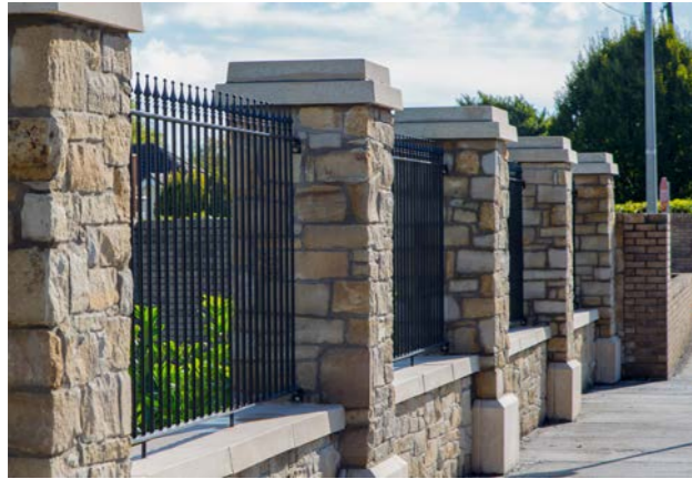
Retaining Butt Wall & Railing 1.8m high
