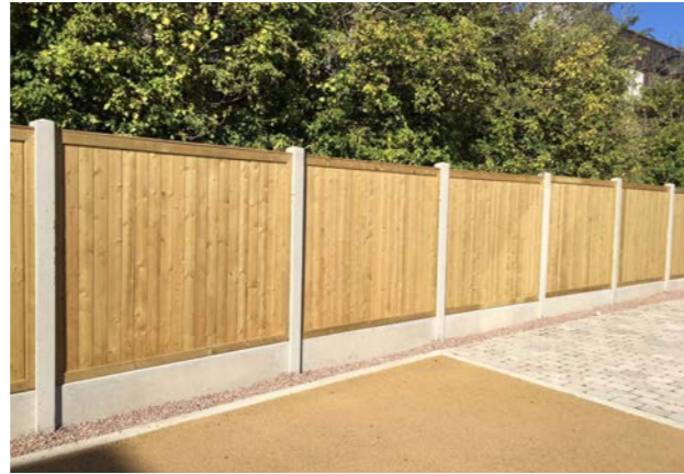
Residential Boundary Fence Timber Panel & Concrete Post Fence █
